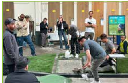
INSTALLATION DEMONSTRATION gives attendees a first-hand look at the proper installation of artificial grass.
